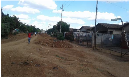
Road needs rehabilitation
