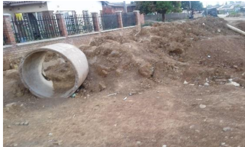
Road needs clearing and rehabilitation
