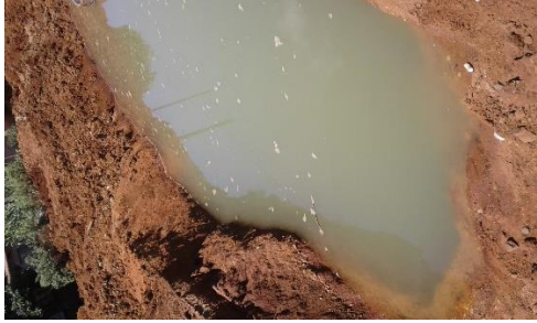
Ground water filled the trenches
