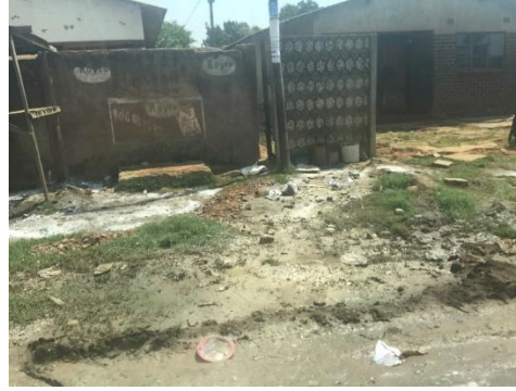
RAW SEWER FLOWING
