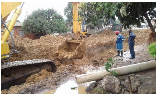
Removing collapsed material
