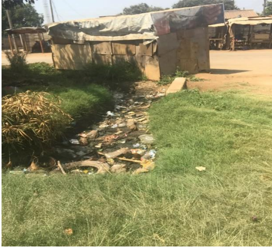
DRAIN FILLED WITH RAW
