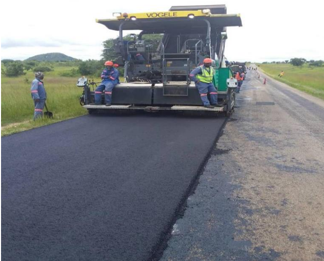
Surfacing in progress asphalt overlay
