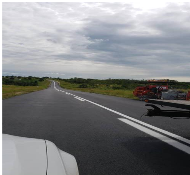
Road marking operation in progress
