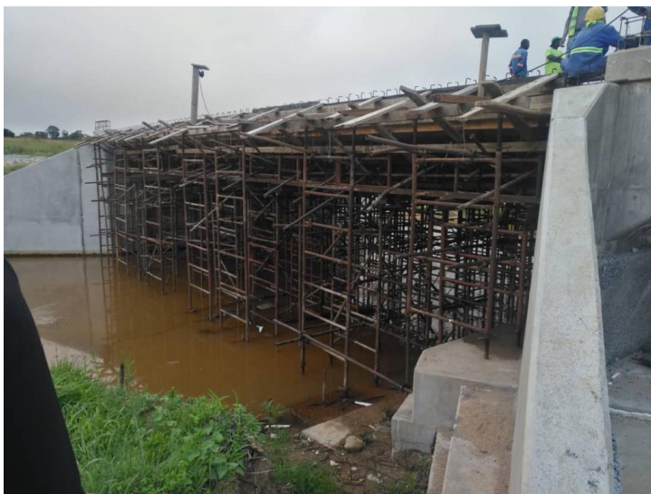
Bridge construction in progress
