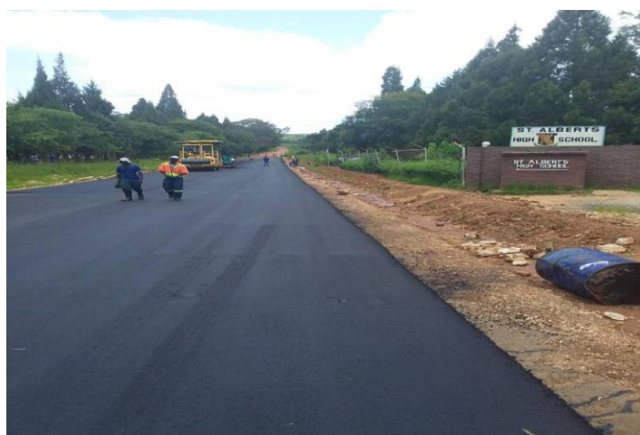
Surfacing in progress 30 mm asphalt overlay
