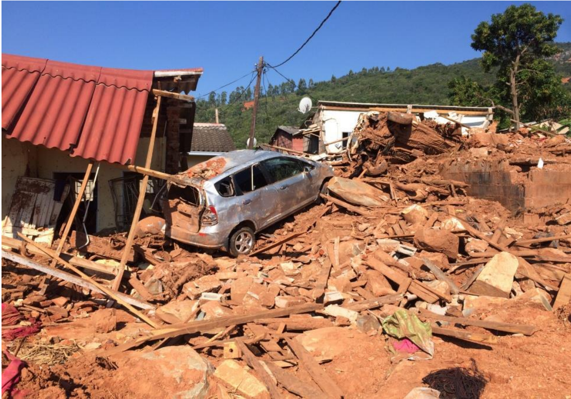
Infrastructure and property destruction
