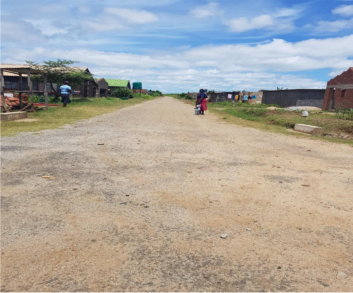
Completed road section on housing project.
