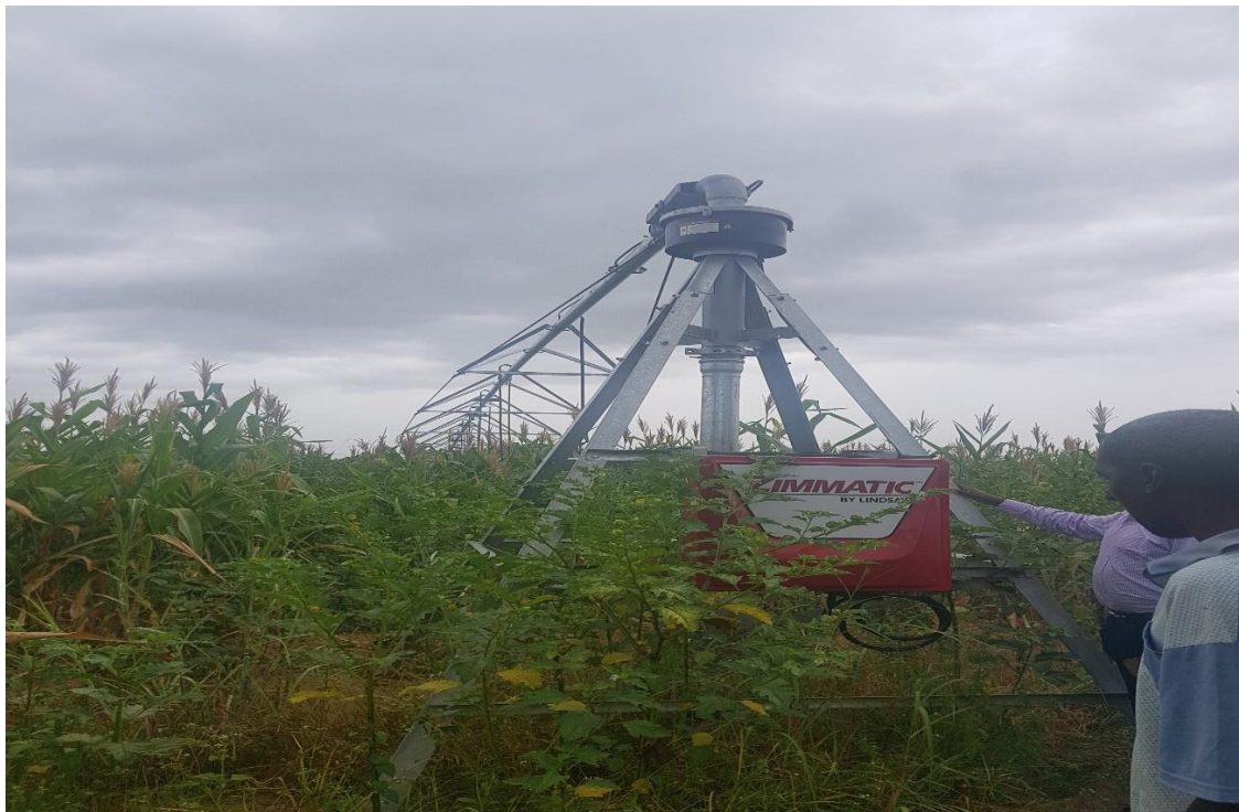
One of the four installed centre pivots
